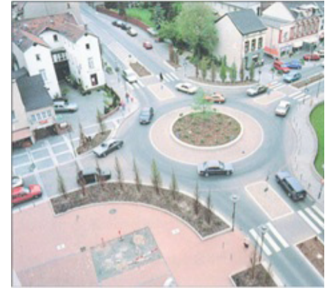
Figure 33: Example of a roundabout in an urban setting
