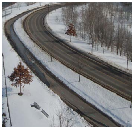
Figure 26: Plowed Bike Trail Next to Road
